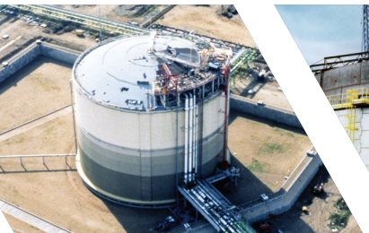
Containment dikes for ammonia tanks - Montoir (France)
